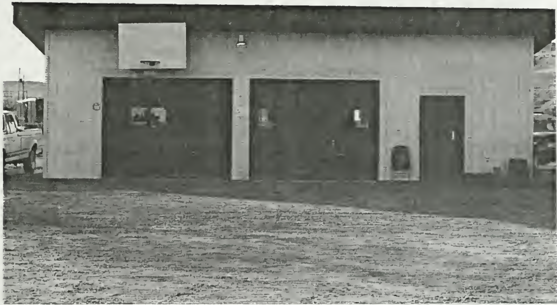
View of maintenance garage.
